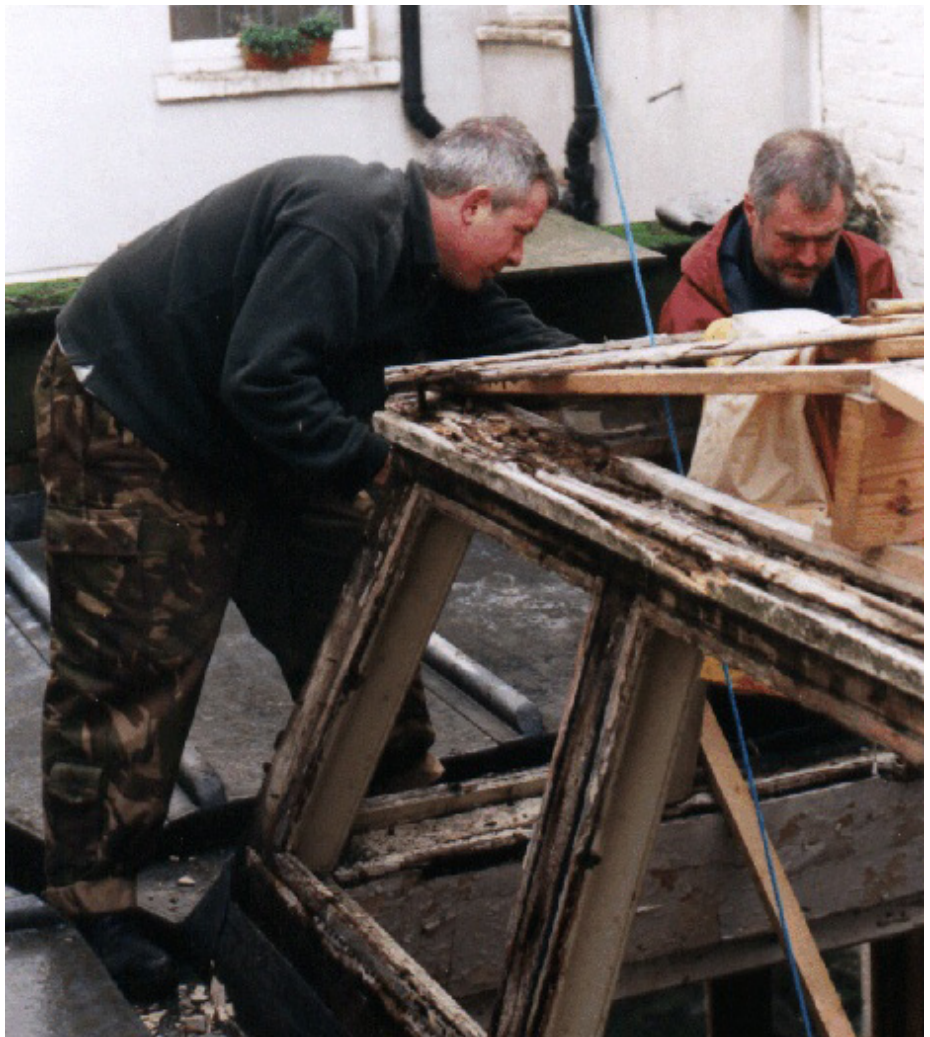
Repairing the skylight at No. 10
