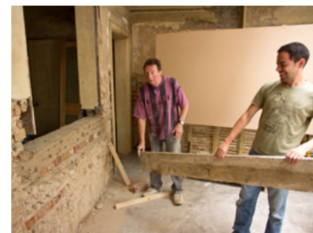
Striking the shuttering several days after the repair has been made.
