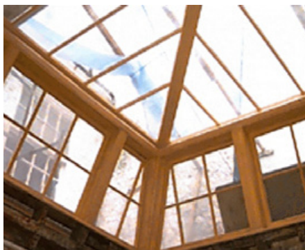
The skylight at No. 10 nearing completion
