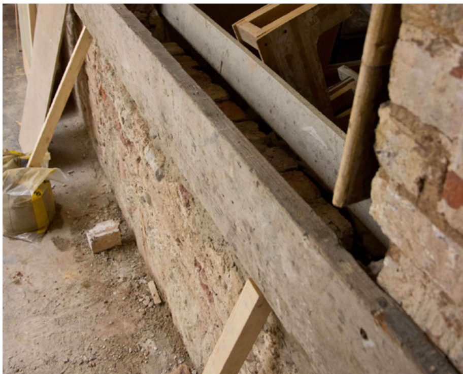
Erecting shuttering at the start of the bungalow repair process
